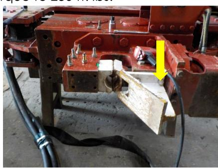
Install short jaw guide (4050359) using the same bolts (9015917) and lock washer (9030610) from the other jaw guide. Torque to 250 ft. lbs.
